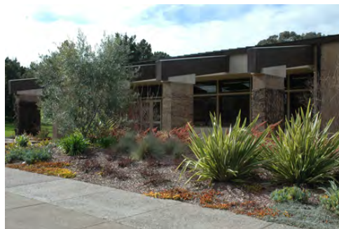
Existing Administration Building
