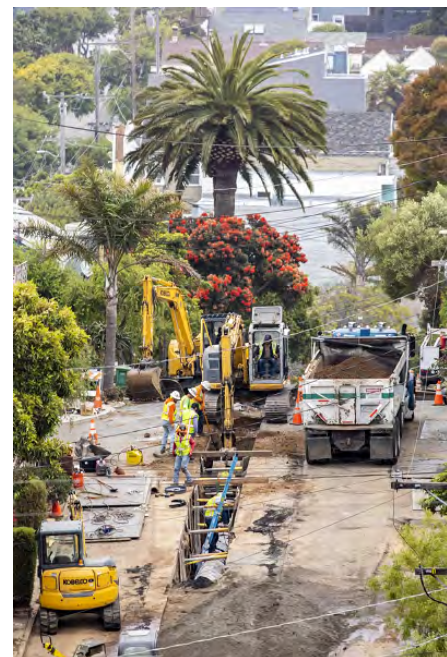
Prospect Avenue Water Main Replacement
