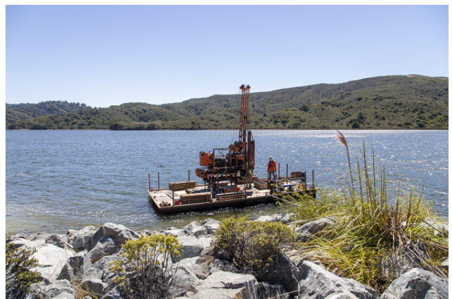
Barge Launch for Geotechnical Drilling in Reservoir
