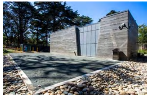
North Lake Well Station
