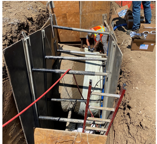
Valve Lot where New Valve will be Installed for Safe Entry
