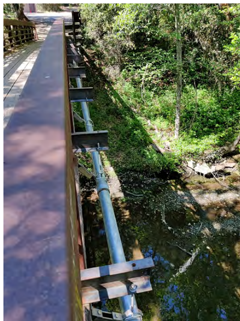
New Water Line Installed on Headquarters Bridge
