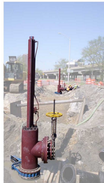
Typical Hot Tap for Line Stop Insertion
