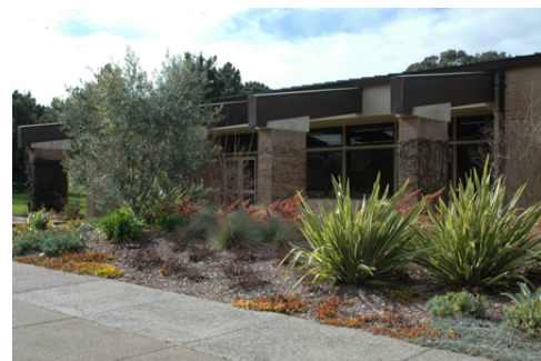
Existing Administration Building
