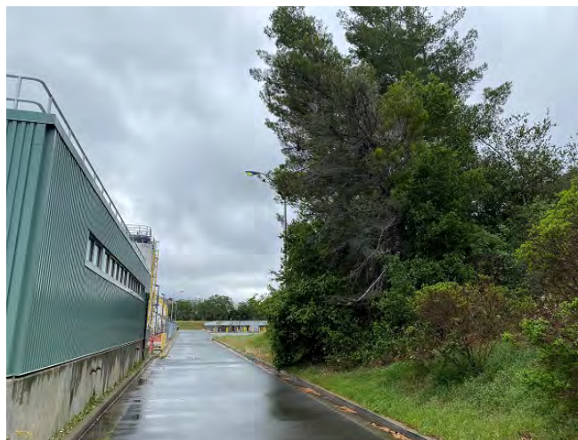
Existing Access Road at Chemical Tanks at SVWTP
