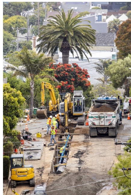
Prospect Avenue Water Main Replacement
