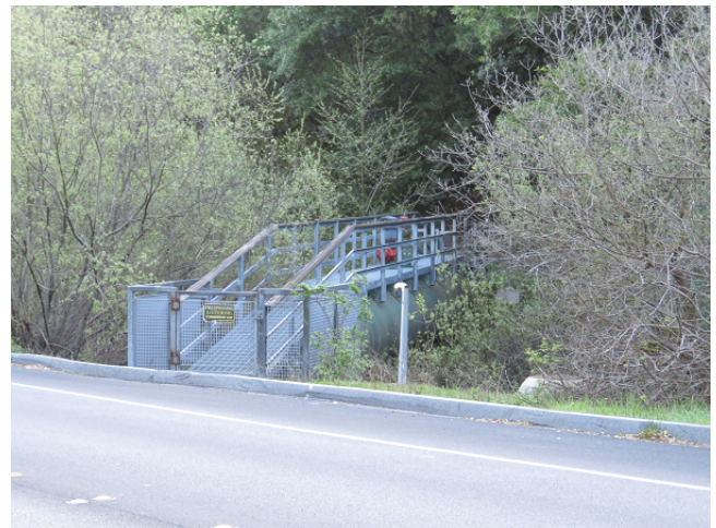
CSPL2 Creek Crossing
