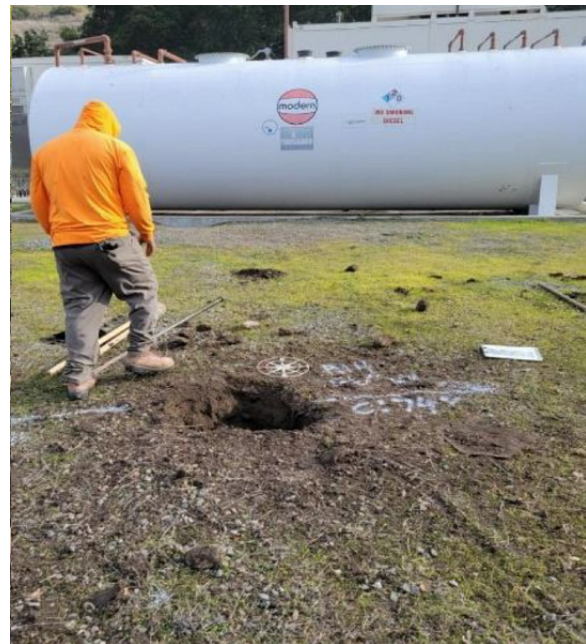
Utility Exploration at San Antonio Pump Station
