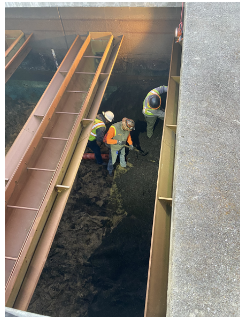
Removal of Filter Media
