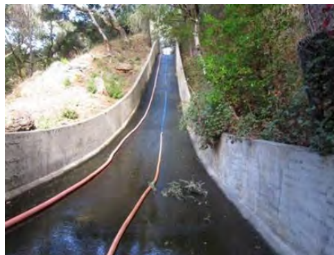
Spillway cleaning and mapping for condition assessment
