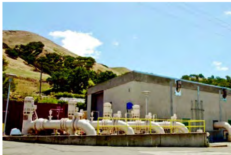
San Antonio Pump Station building looking southeast
