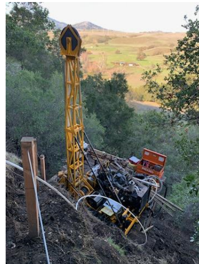
Helicopter Boring Equipment
