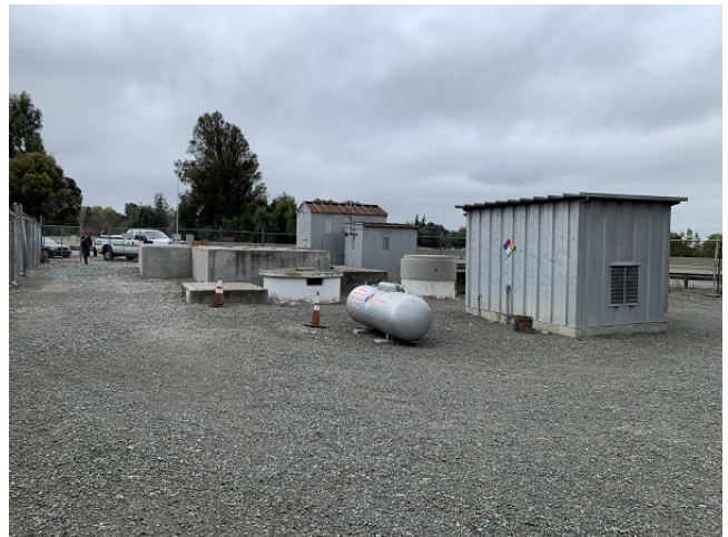
Valve Lot where New Valve will be Installed for Safe Entry
