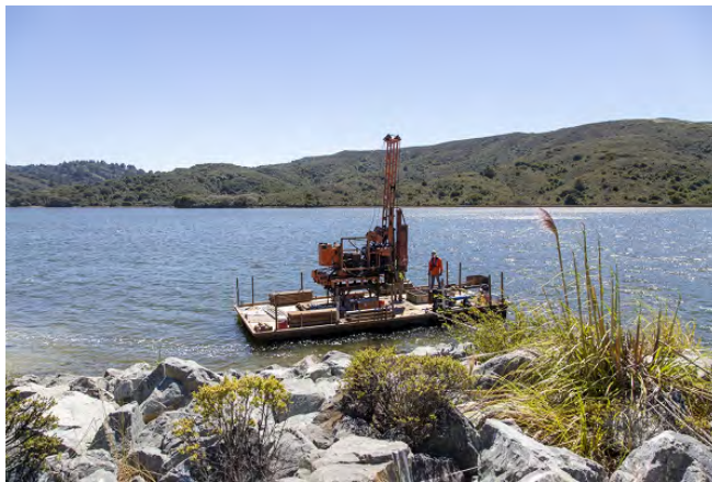
Barge Launch for Geotechnical Drilling into Lake
