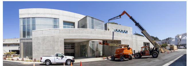
Exterior of Buildings 580 and 581
