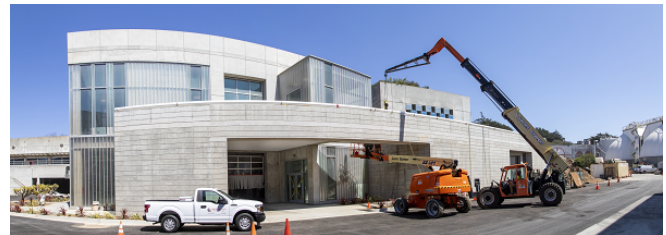
Exterior of Buildings 580 and 581
