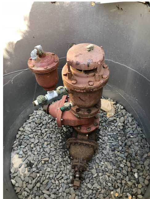
Typical Appurtenance to be Upgraded
