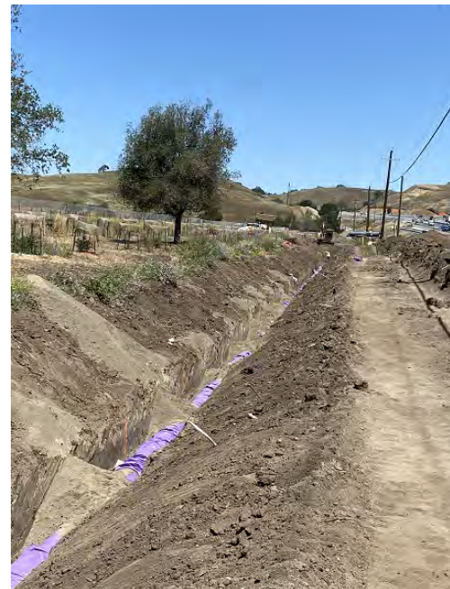
Installation of pipeline by Highway 680
