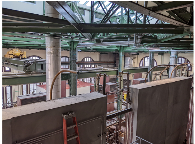
Roof installation of Pump Station No. 2
