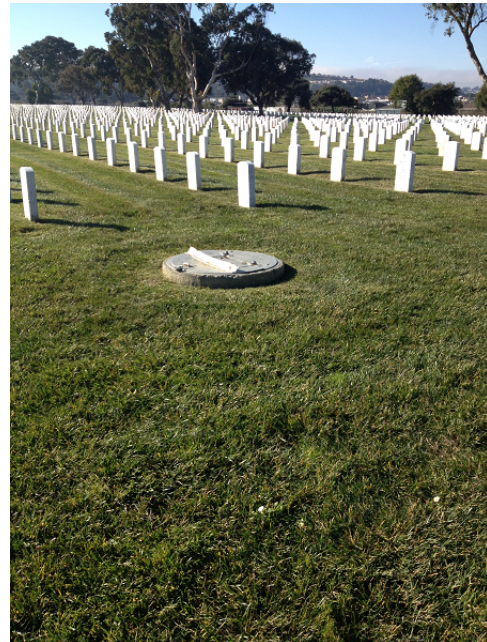
Typical Appurtenance to be Upgraded
