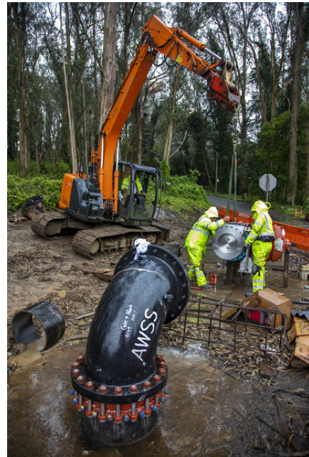
Installing valve number No. 2 for the Clarendon Supply Project
