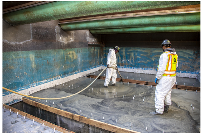
Placement of Leveling Grout in Filter Box
