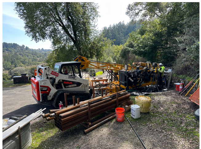
Right Abutment Horizontal Drilling Operation
