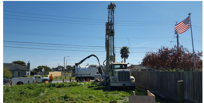
Typical Anode Well Drilling
