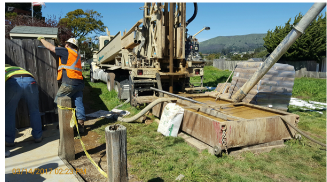
Drill Rig Photo
