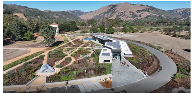
Aerial view of the project site
