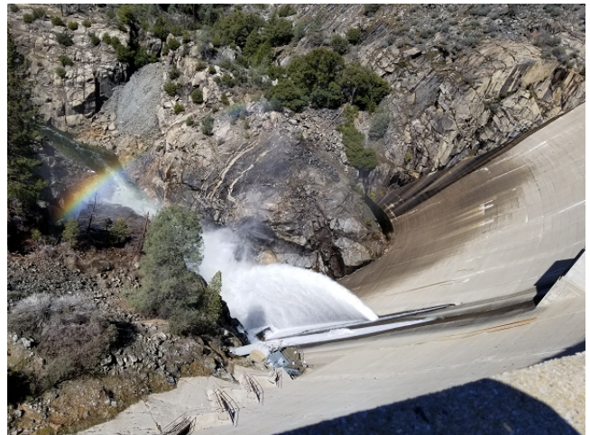
O'Shaughnessy Dam Outlet Valve Release
