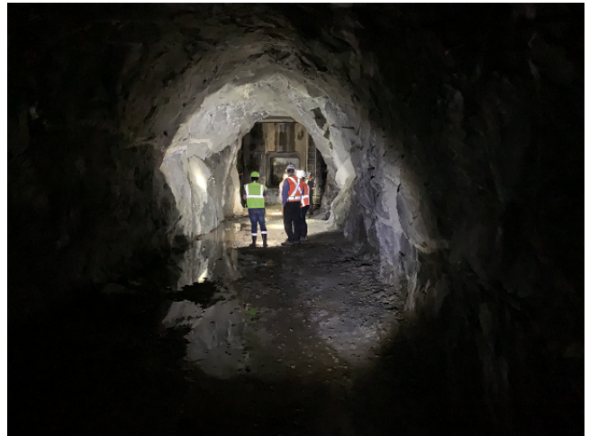
Inside Hetchy Adit to Evaluate Geologic Condition of the Proposed Bulkhead Location
