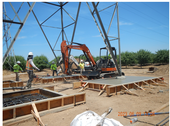
Rebar and Foundation Pour at Structure 571S [HH-1007]
