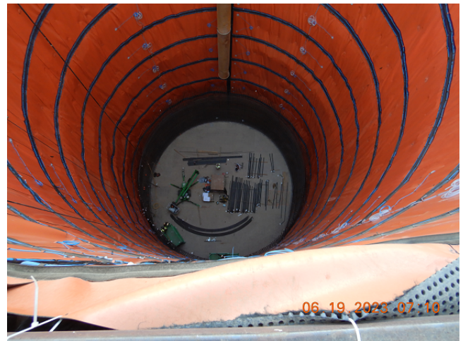
Completed waterproofing in Flow Control Facility shaft
