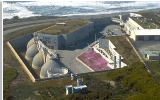
Oceanside Treatment Plant
