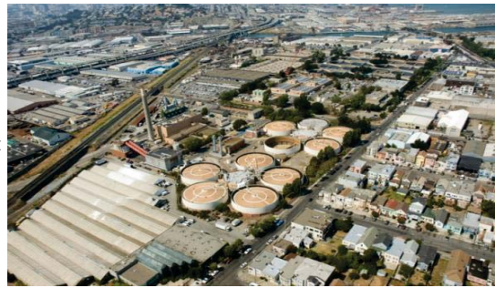
Southeast Treatment Plant
