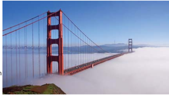
Fog on Golden Gate Bridge
