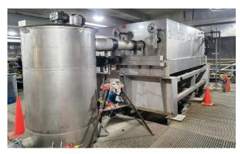
Proposed New Rotary Drum Thickener (RDT) and Associated Flocculation Tank Assembly
