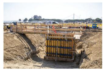
Installing Formwork for Concrete Placement of Influent Pumping Structure Walls
