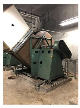
Existing Exhaust Fan Assembly Identified for Replacement at Building 011 Exhaust Fan Room.
