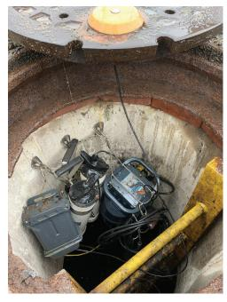
Existing Field Instrumentation Equipment Installed In a Sewer Manhole
