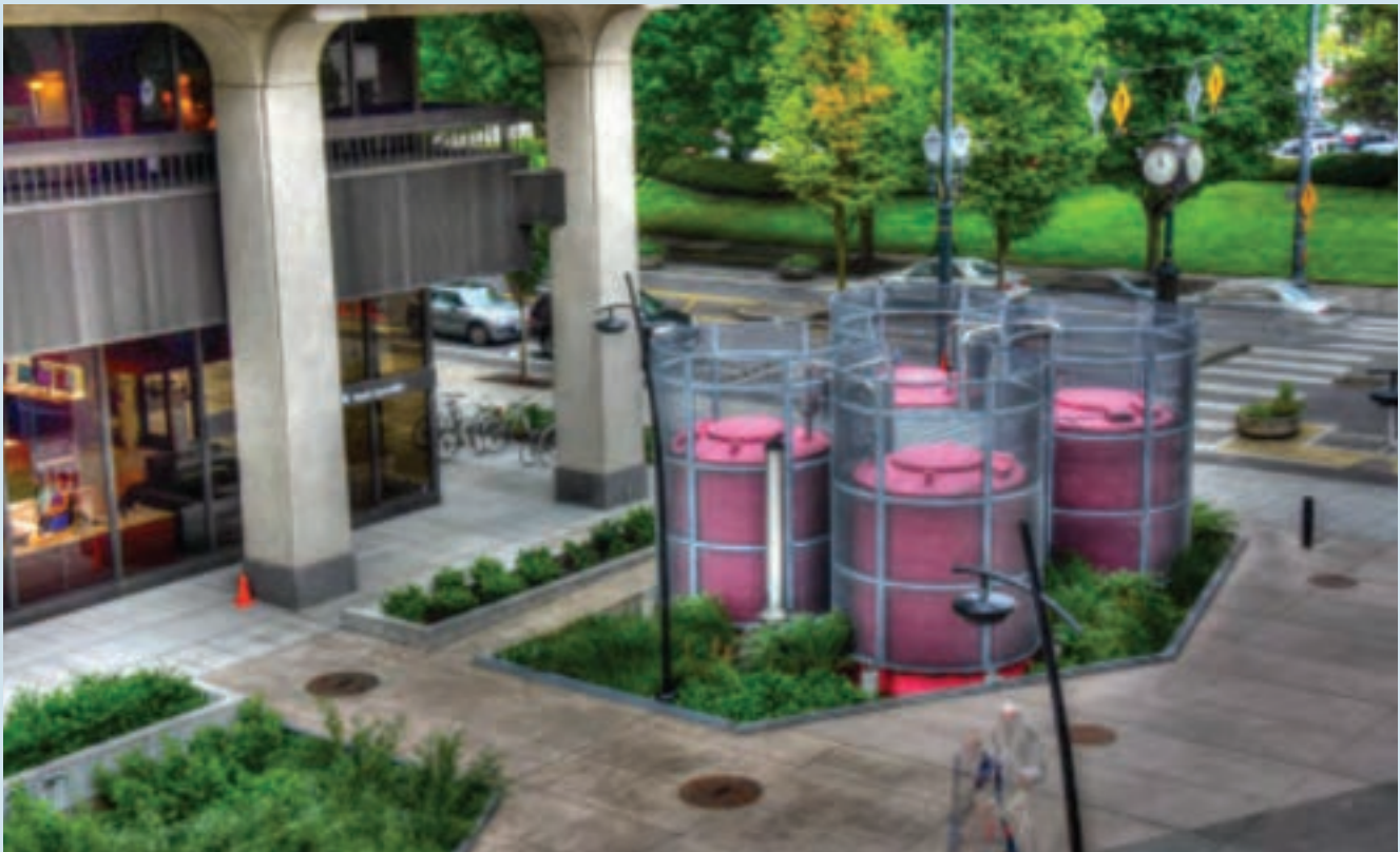
Hassalo on Eighth Wastewater Treatment System (image courtesy of Jim G. Maloney/Biohabitats, Inc.)
