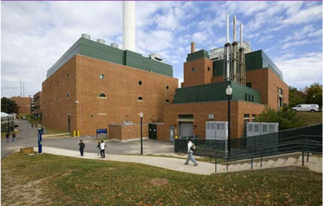
UConn Central Utilities Plant
