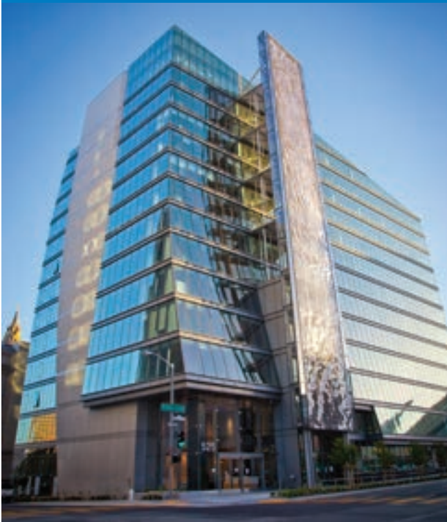
San Francisco Public Utilities Commission Headquarters
