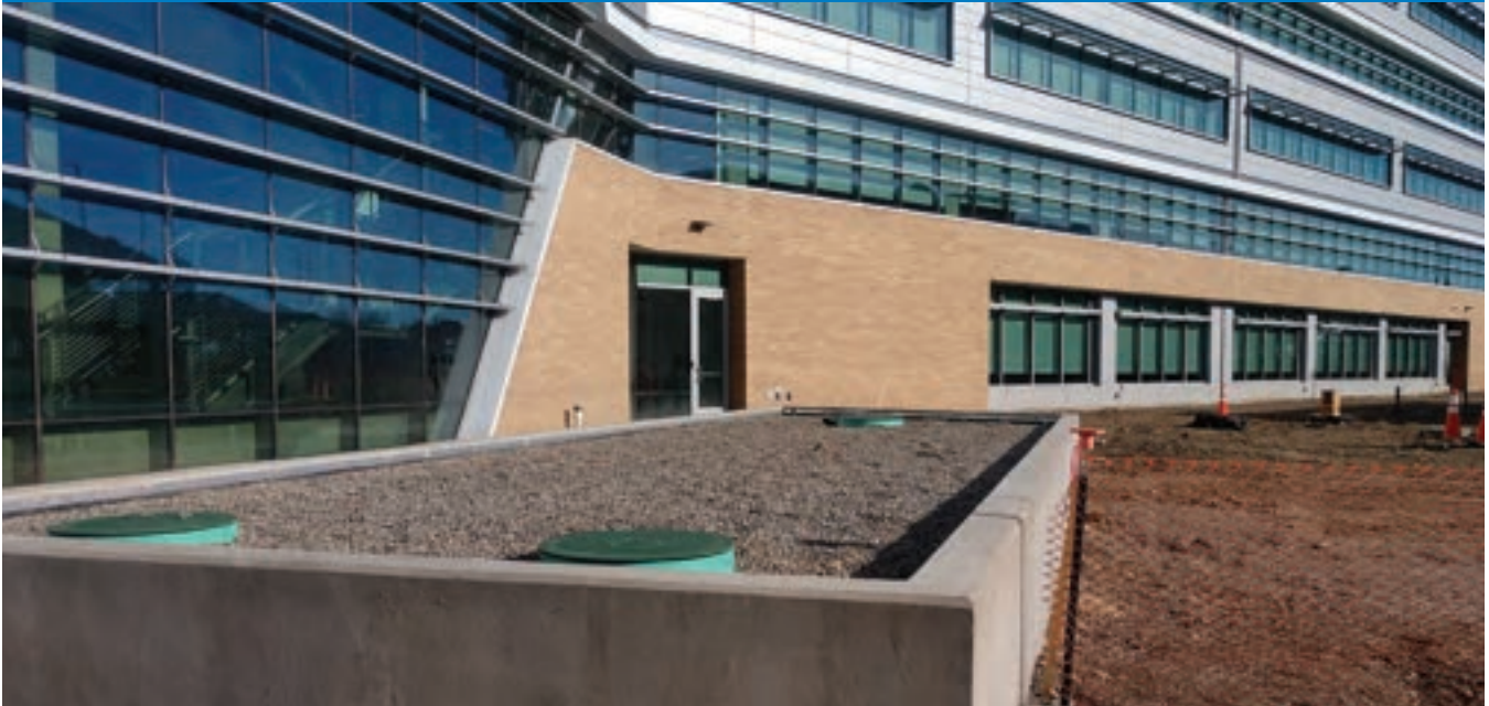
3rd stage of wetland treatment during its construction on the roof (Image courtesy of Denver Water)
