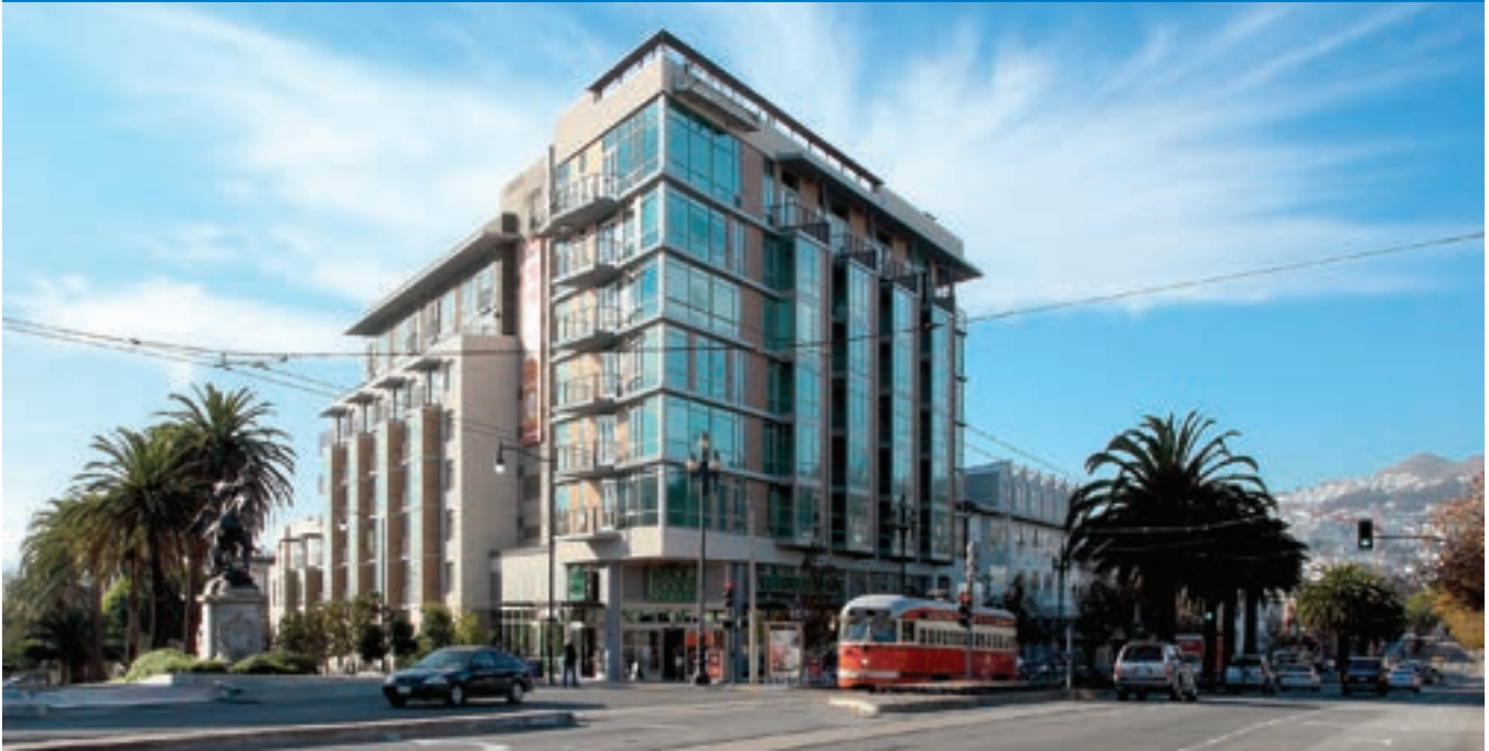
38 Dolores Street (image courtesy of BAR Architects)
