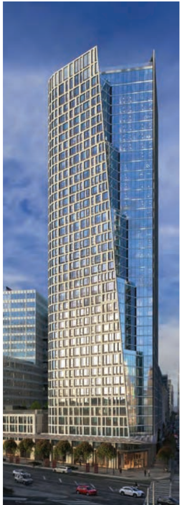
Fifteen Fifty, a high-rise residential tower in San Francisco, CA is reusing graywater and rainwater for toilet and urinal flushing and irrigation. (image courtesy of Epic Cleantec)
