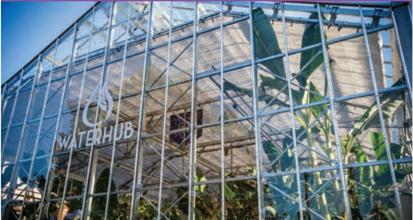
Exterior of the WaterHub greenhouse at Emory University (image courtesy of Sustainable Water)
