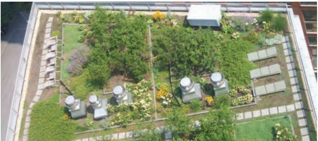
The green roof reduces runoff, insulates the building, and is irrigated by the onsite reuse system (image courtesy of NSU)
