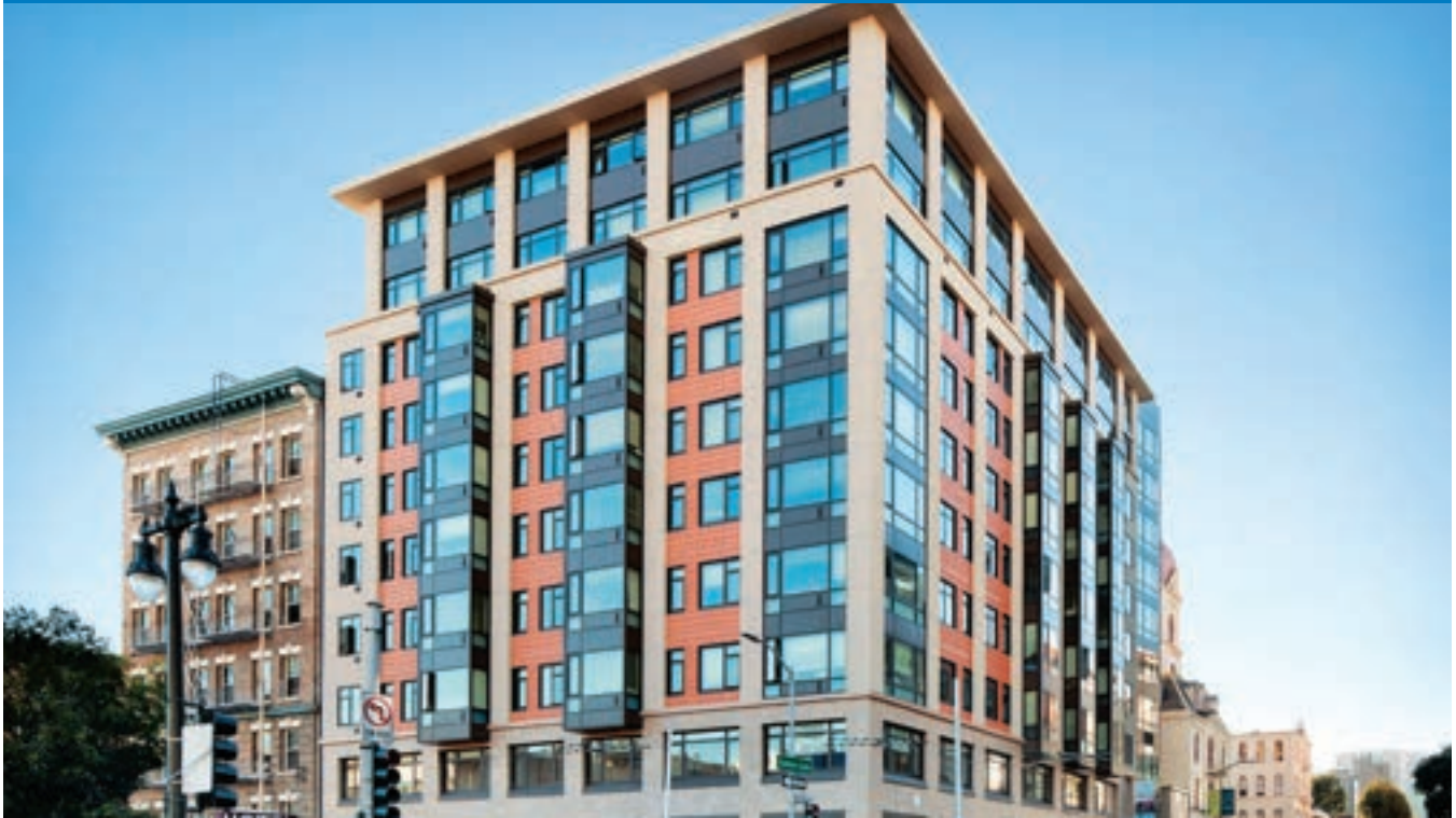
The Vera Haile Housing and St Anthony's Foundation Dining Room and Social Work Center (image courtesy of David Wakely Photography)
