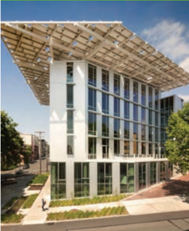
The Bullitt Center (photo by Nic Lehoux)
