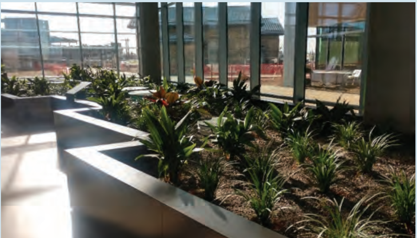
Denver Water's Wetland System Treating the Building's Blackwater in Denver, CO (image courtesy of Denver Water)
