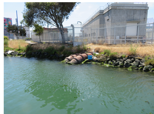
Current pipeline crossing at Islais Creek
