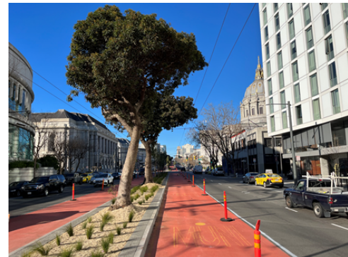
Sewer Completion along Van Ness
