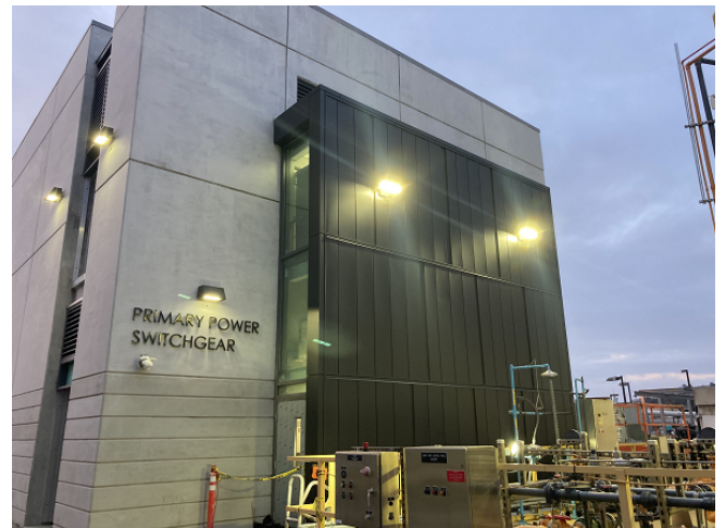
West Side View of Primary Power Switchgear Building
