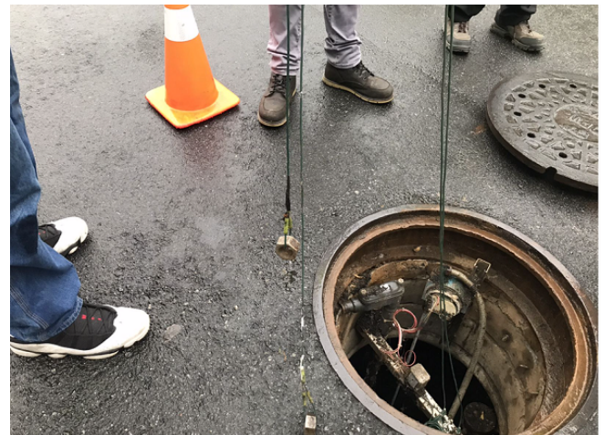
Project team performing field measurements and investigation.
