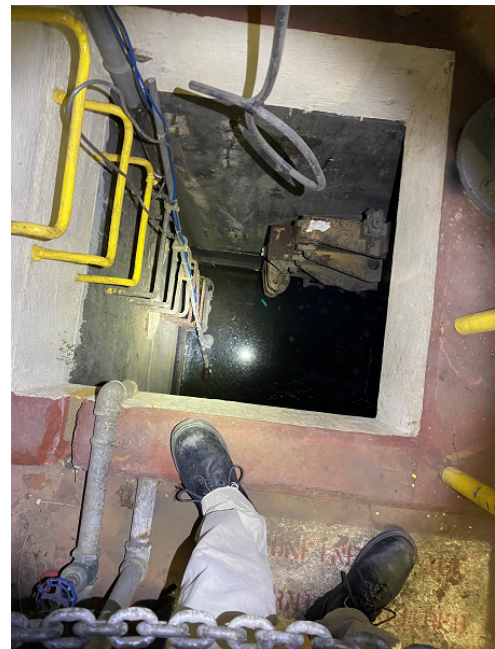
Entrance to Geary Underpass Pump Station
