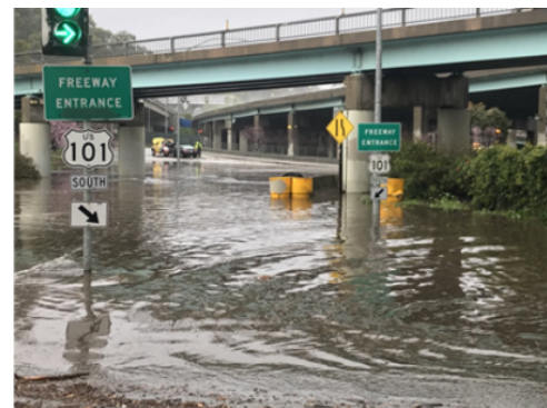
Flooding at the I-280/Hwy 101 interchange at Lower Alemany area, during the rainfall of February 13, 2019
