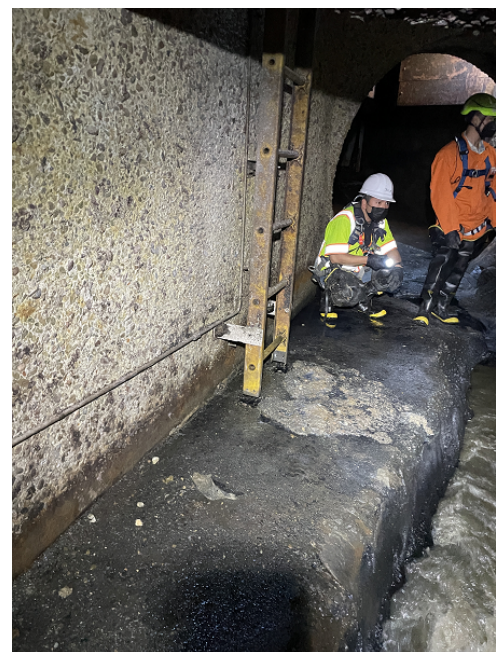
Howard CSD inspection after cleaning.
