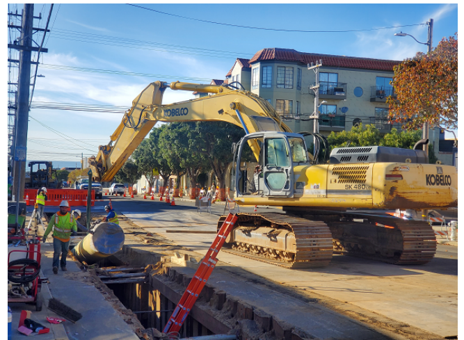
Installation of 36-inch steel pipe
