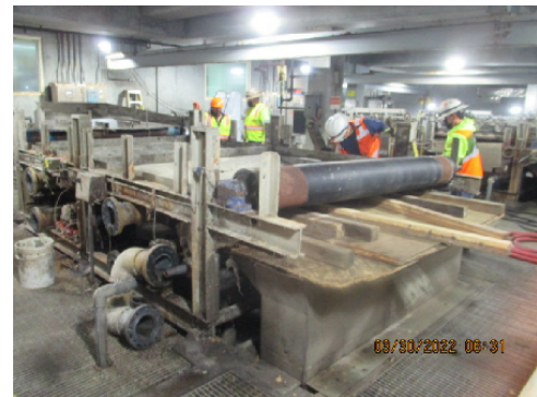
Selective equipment demolition to GBT No. 1; this work is expected to be completed prior to the project contract work commencing on the replacement of GBT No. 2 and GBT No. 3.
