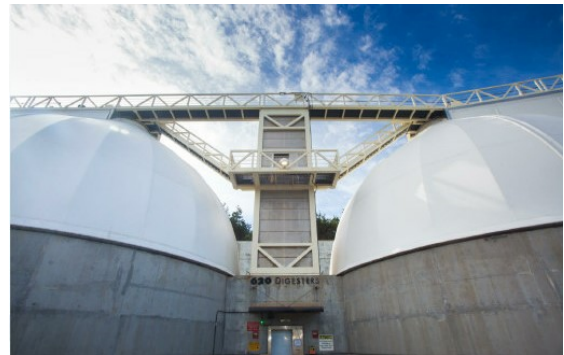
Contract A; OSP 620 Elevator is subject to modernization under the project.
