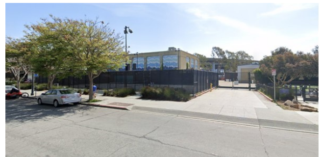
Channel Pump Station
