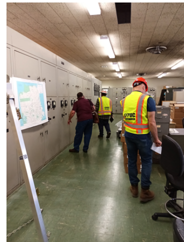
WWE staff and design team surveying existing obsolete electrical equipment at NPF 930 Administration Building.
