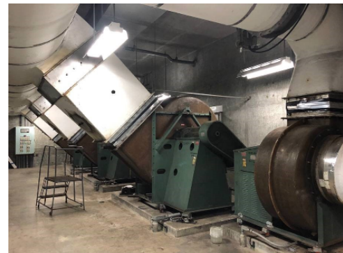
OSP Building 011 as-found condition of ventilation exhaust systems
