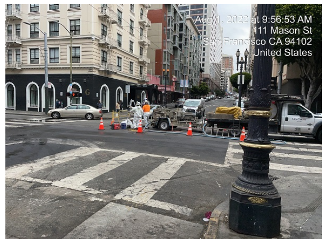
Contract B: Spray Mortar Installation (WW-712).
