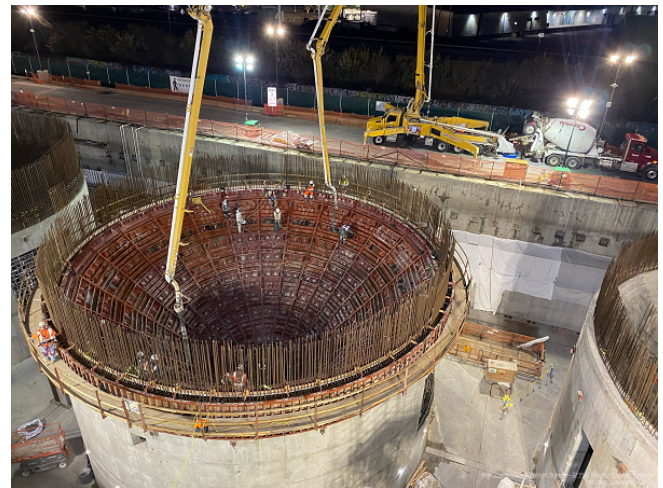
Placing Concrete in Tank 4 Hopper
