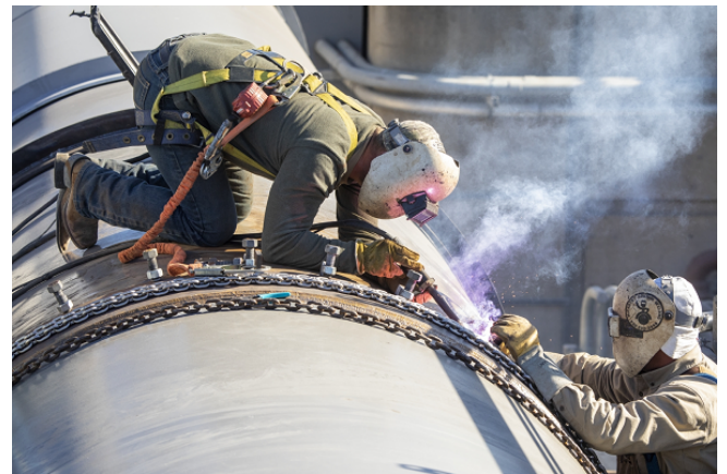
Installation of final piece of 84in SR pipe
