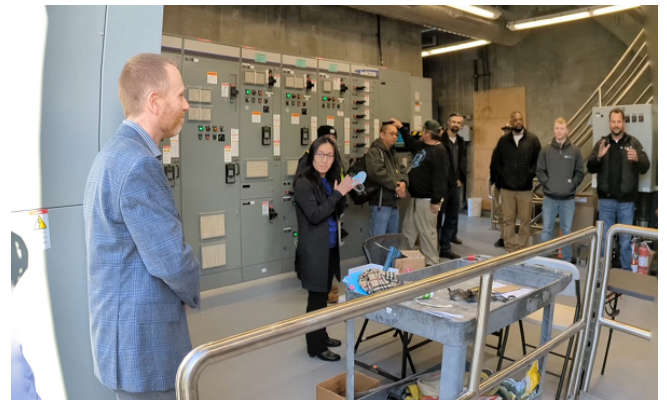
On December 6, 2022, the project team and contractor gathered at the pump station to celebrate the successful completion.
