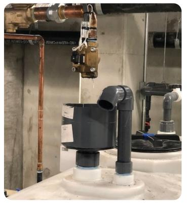
Potable make-up water is supplied to the treated water storage tank via an air gap.
