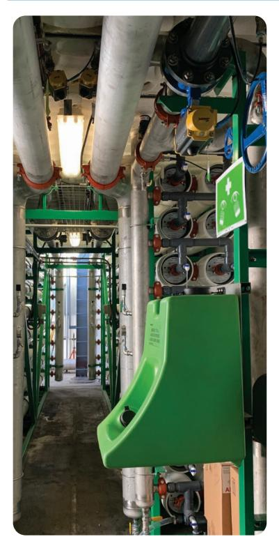
Energy Center San Francisco captures foundation drainage from Powell Street station and redirects it to their District Energy Plant nearby for producing steam. The plant has an eye wash station for the safety of all personnel working on the onsite treatment system.
