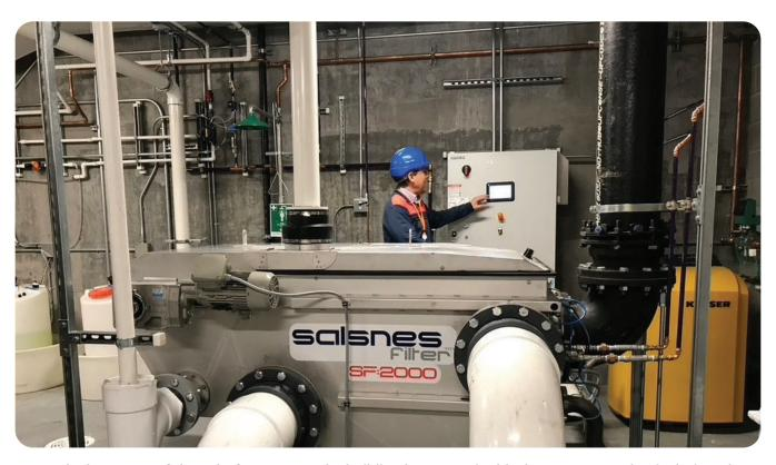
In the basement of the Salesforce Tower, the building has an onsite blackwater system that is designed to capture all of the building's wastewater, treat, and reuse it for toilet flushing and drip irrigation.
