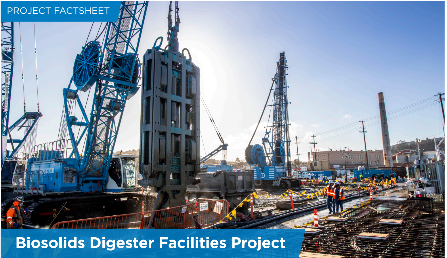
Pictured above: Biosolids Digester Facilities Project Construction
