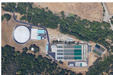
Aerial view ng SVWTP
