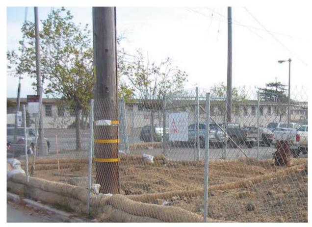
Erosion control blankets are being used to stabilize disturbed soil area.
