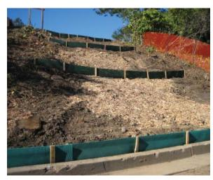
Plastic mesh fencing is installed parallel to the contours along the slope.
