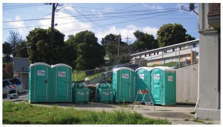
Properly installed portable sanitary facilities.
