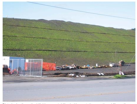
Disturbed soils on the hillside were stabilized with vegetative growth and fiber rolls.
