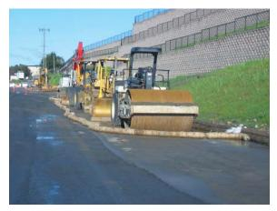
Inactive paving equipment is properly stored with perimeter protection.
