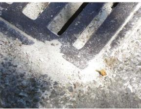
Runoff containing concrete admixtures from unprotected construction activities have made their way to a drainage inlet.
