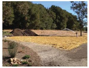
Water is applied to exposed soil and stockpiles to prevent dust generation.
