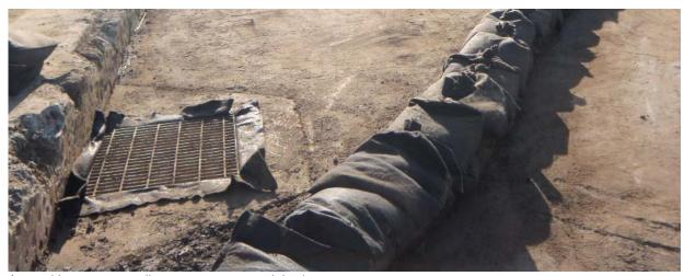
A gravel berm acts a sediment trap near a catch basin.
