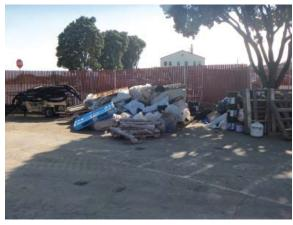
There are no dumpsters, containers or diversion structures to stop stormwater runoff from coming in contact with this construction litter and debris.
