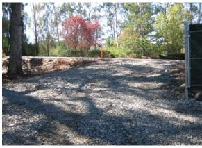
The contractors properly installed a stabilized construction roadway.
