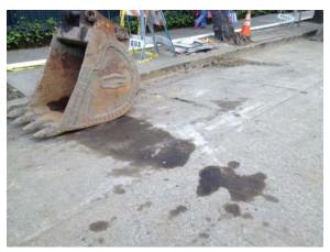
Minor oil spills need to be cleaned to prevent them from running into the storm drain system.
