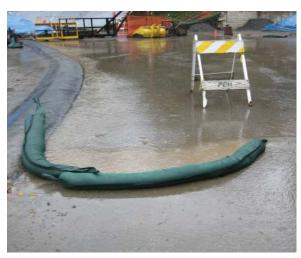
Gravel bags are used to form a check dam along the roadway.
