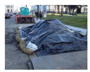
Asphalt debris is escaping from this poorly installed stockpile. Asphalt can release pollutants like hydrocarbons when not properly contained.
