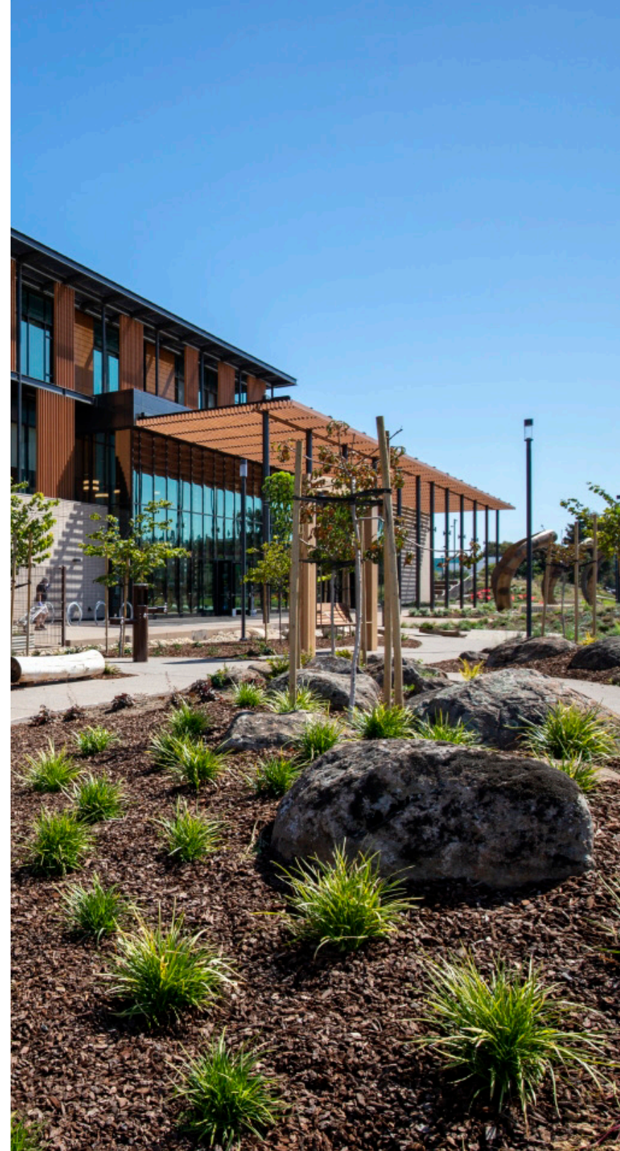
Southeast Community Center
