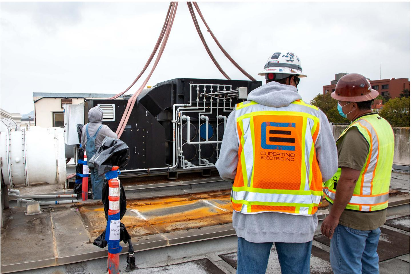
*North Shore Pump Station Wet Weather Improvements: Removal of two Odor Control Units from the roof of the North Shore Pump Station.*
