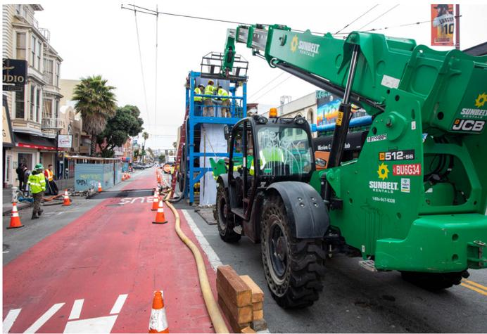
*Mission Street, 16th to Cesar Chavez, Brick Sewer Rehabilitation Project: The project uses a trenchless method called cured-in-place pipe (CIPP) technology to rehabilitate the brick sewer tunnel.*
