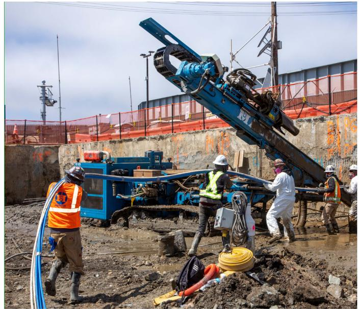
*Crews of the Biosolids Digester Facilities Project at the Southeast Treatment Plant install tiebacks along the retaining wall for the new Digester Facilities to anchor and reinforce the structure.*
