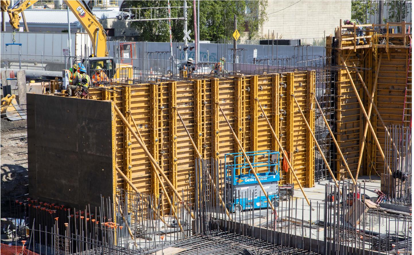
*Southeast Wastewater Treatment Plant (SEP), Headworks Facility Project: Concrete pour on wall in Grit Tank Area 45.*
