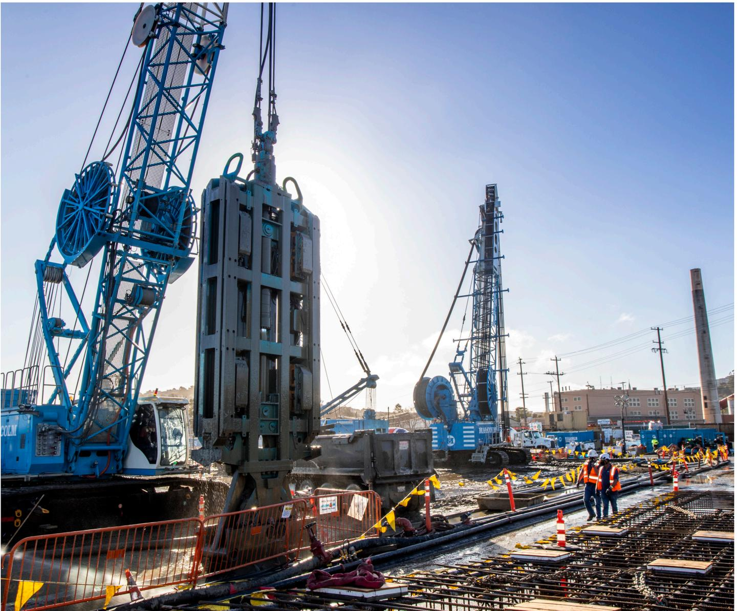
*Southeast Wastewater Treatment Plant: Biosolids Digester Facilities Project: Clamshell Grab Machinery, used for slurry wall excavation.*
