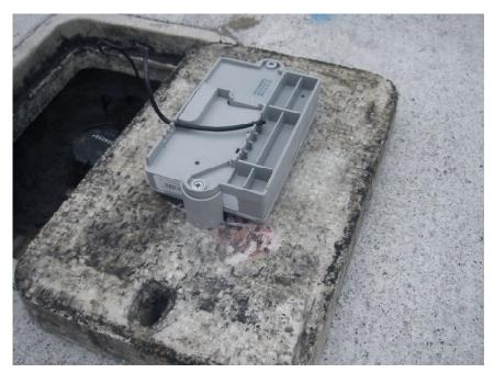
Top: Water meter with transducer.
