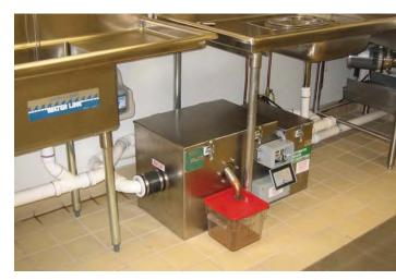
**Figure 4.** Example of an installed automatic grease removal device. Source: The Wastewater Solutions Update
