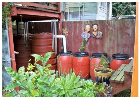
Projects can install a tank or cistern that collects roof runoff and stores it for indoor or outdoor uses such as irrigation. Roof runoff can be directed to a cistern to capture and detain the design storm volume, and release runoff volume through a low-flow orifice.
